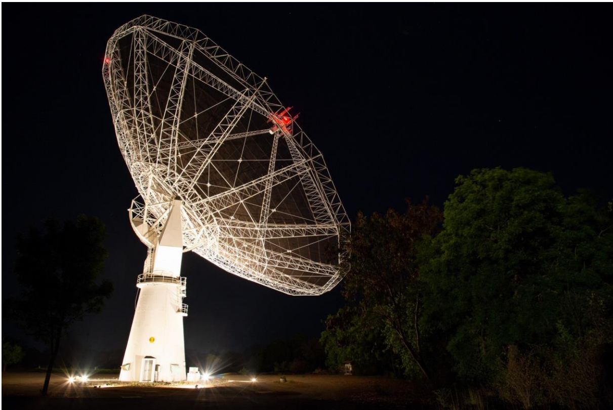
Caption: A GMRT antenna at night. Picture by Rakesh Rao.
