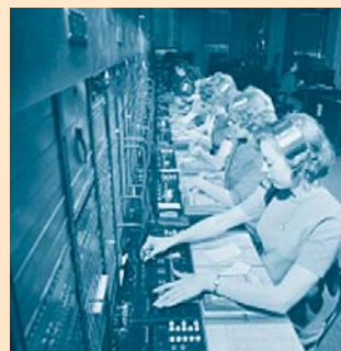
Manual Telephone Exchange
