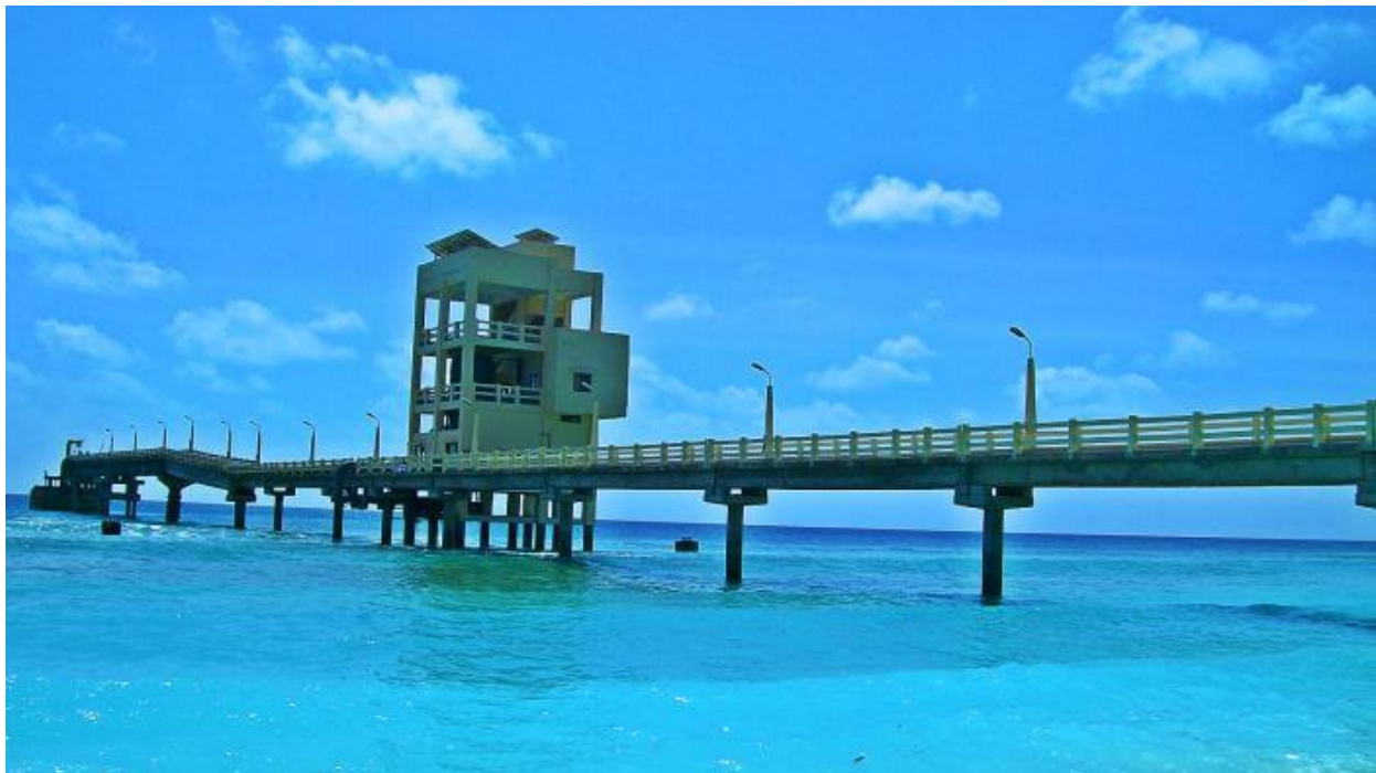
Figure: NIOT desalination Plant
