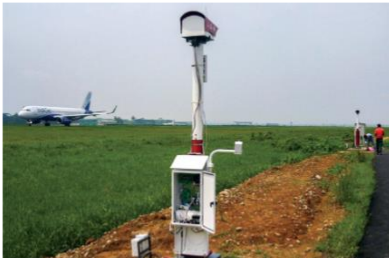
Drishti Transmissometer installed for India Meteorological Department at KIA Airport, Bengaluru
