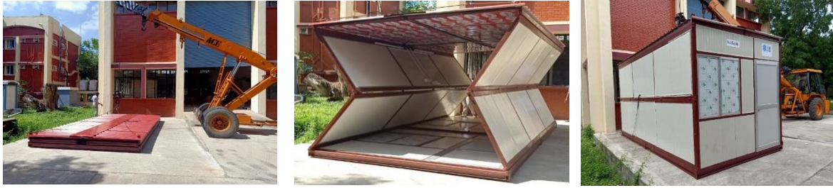
Folded position, Un-folding using crane and ready-to-use PoliTal-M Module
