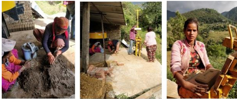
Women's Unit – Compressed Stabilised Earth Blocks at Baaai, Uttarkashi
