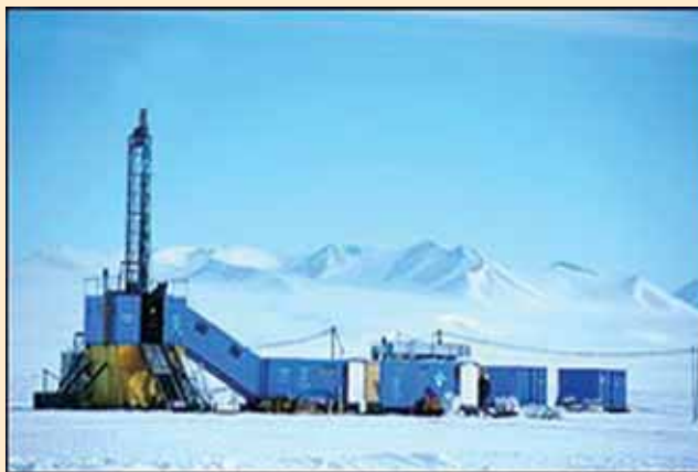
Figure 2: Drill working at Dome-C
