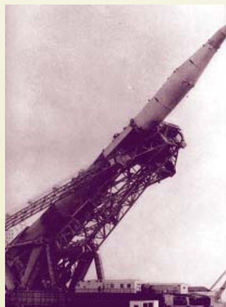
R7 rocket hoisted into launch pad
