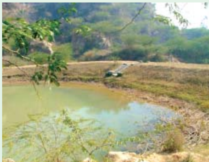
Figure 2: Silt detention earthen structure
