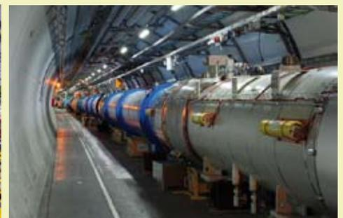
*Beam loss monitors (yellow tubes) installed on
