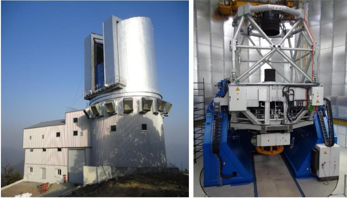
*Figure 7: (a) Building of the 3.6 meter telescope and (b) A fully assembled 3.6m DOT in its dome at Devasthal.*
