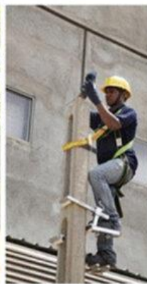
Concrete Pole Climber
