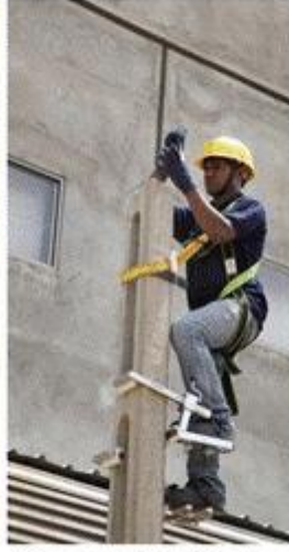
Concrete Pole Climber
