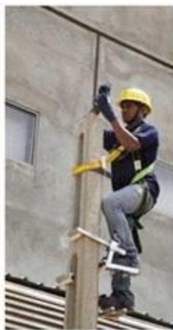
Concrete Pole Climber
